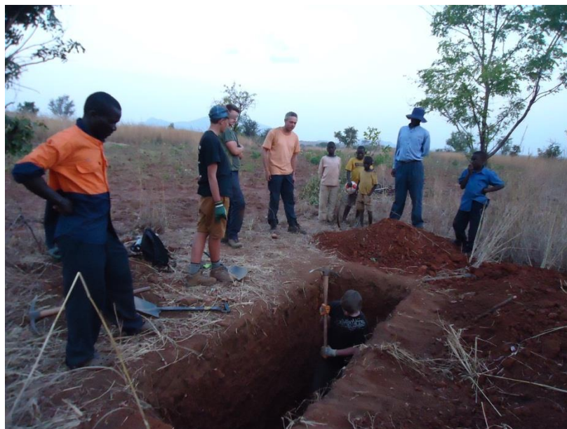
Finishing off the second toilet pit.
