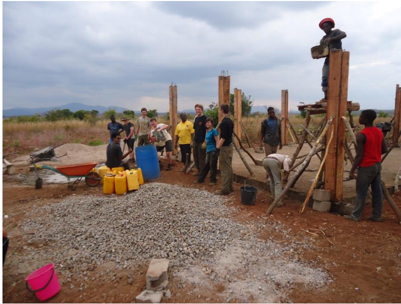
Filling in pillars with concrete.
