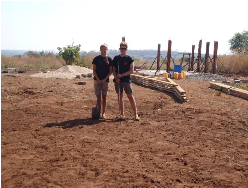
Preparing a playground next to the school building.
