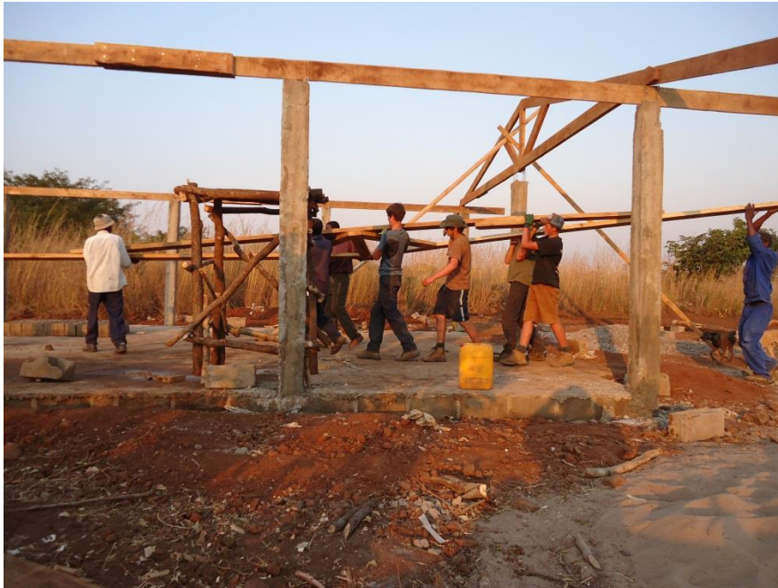
Putting up the roofing trusses.
