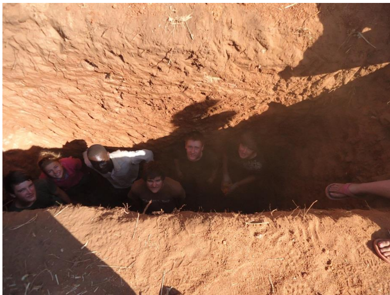
Inside the finished toilet pit.
