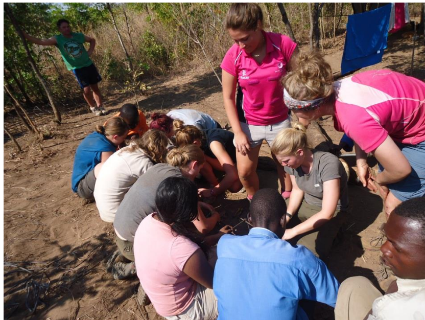
Making frames for the concrete pillars of the building structure.
