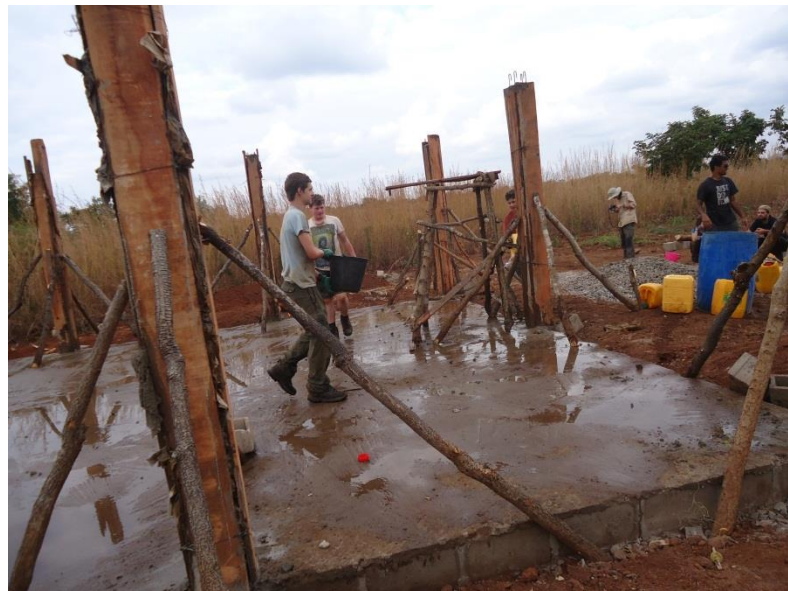
Watering the concrete slab to harden it.
